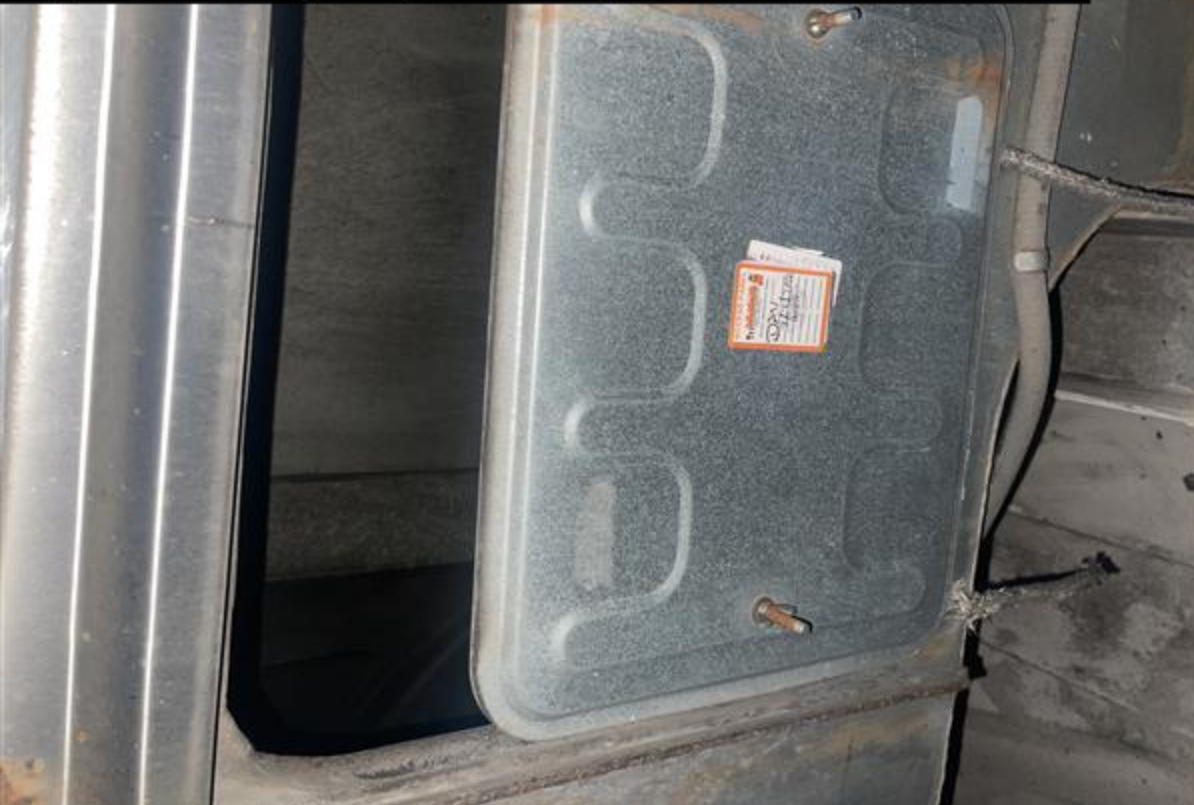
this shows how I found the access panel on the roof. gasket is torn and i was able to re-seat the panel
