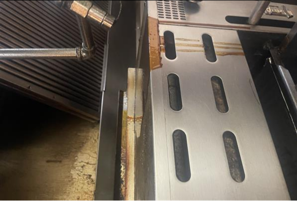
drips from duct onto the oven.
